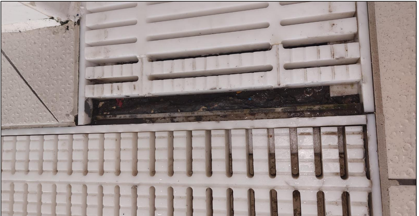
Photo 21: Missing overflow channel – tripping hazard
