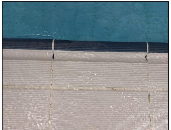
Photo 23: grout missing around poolside (1%)
