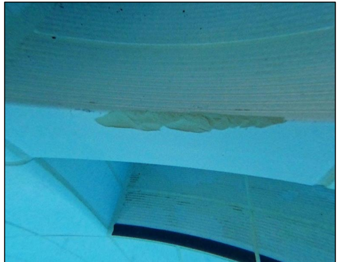
Photo 2: Close up of chipped step tread
