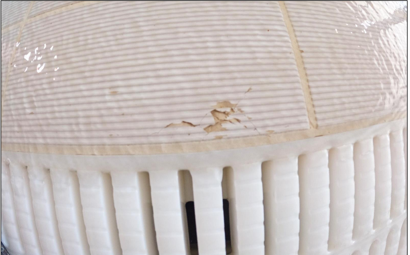
Photo 30: 1 single tile with defect on poolside surround
