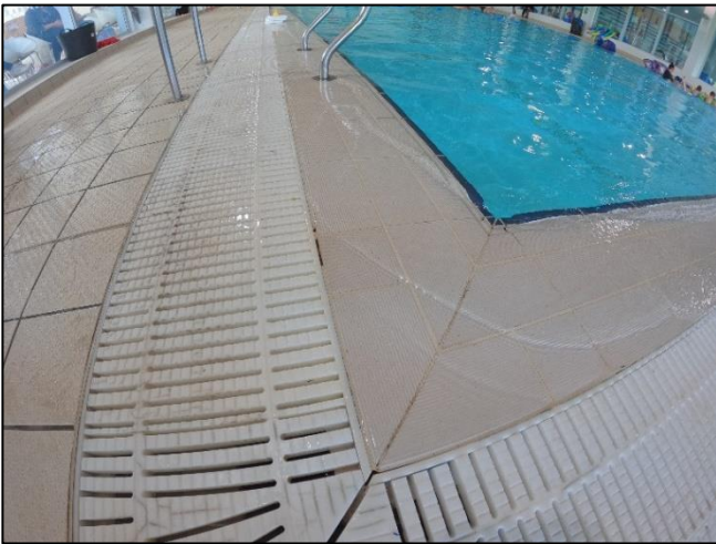
Photo 33: Overflow channel grating in good condition
