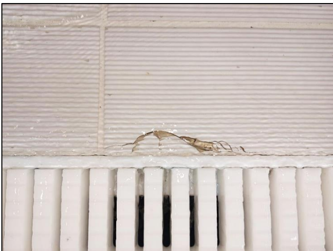
Photo 19- Splintered tile – sharp edges exposed
