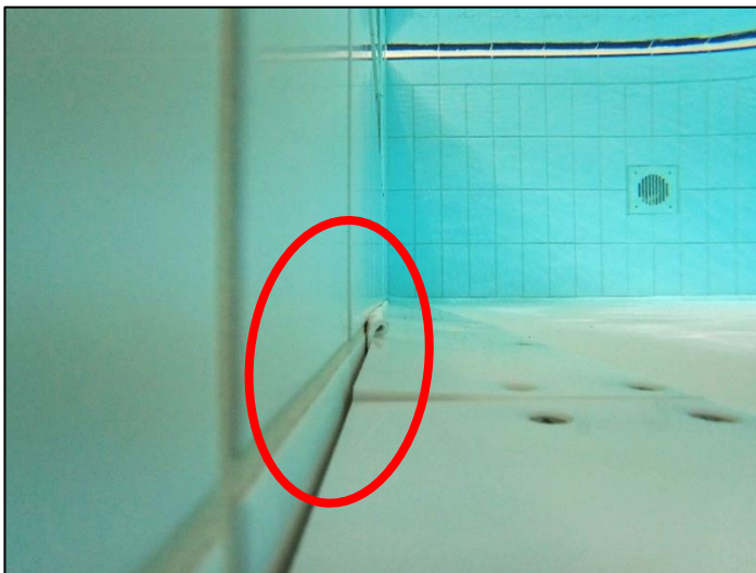
Photo 28: P strip squashed and missing
