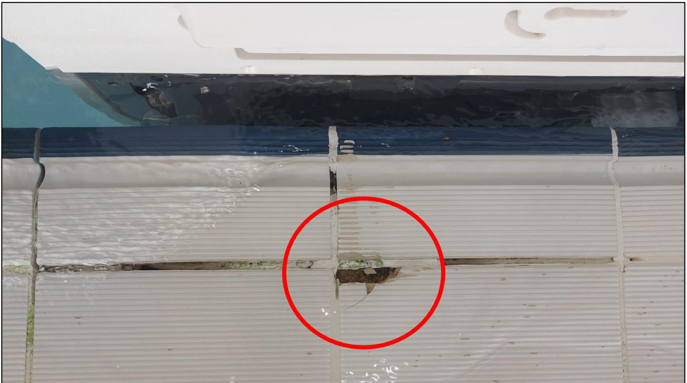
Photo 18: Damaged tile adjacent to hand grip tile alongside the boom
