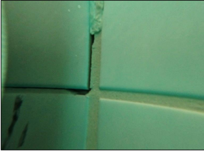
Photo 9 – Missing grout next to boom on wall
