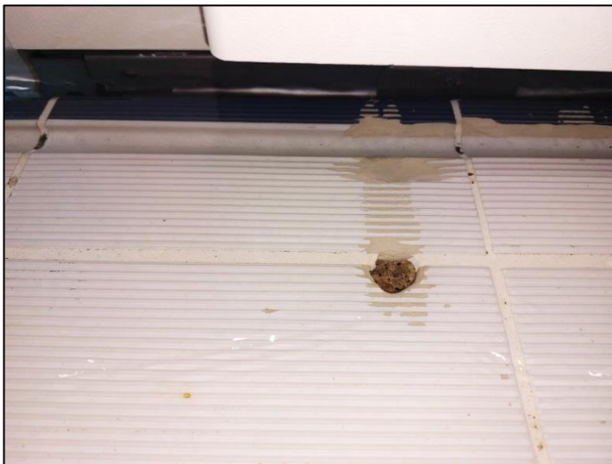
Photo 22: Hole within pool surround tiling
