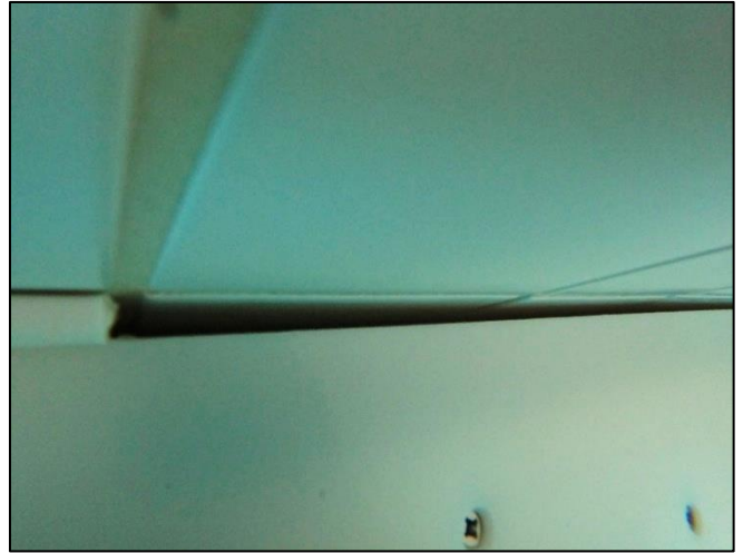
Photo 27 – Missing P Strip – gap exceeding 8mm
